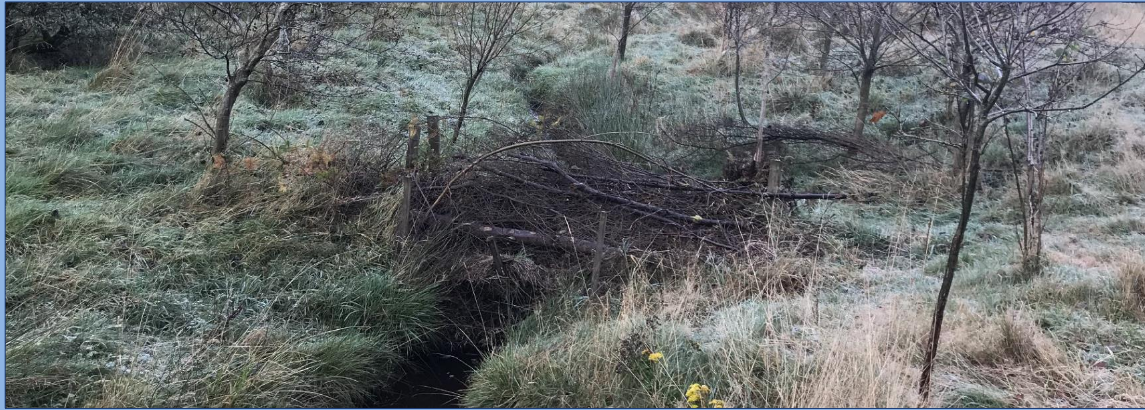
Figure 1: Leaky dams can slow the flow of water by storing it on the floodplain.
