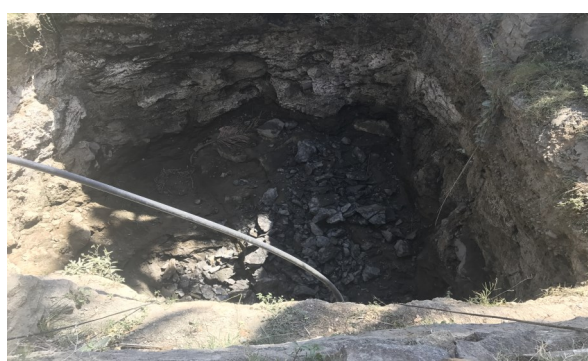
Figure 5: Farmers deepening the dugwell in the coconut farm
