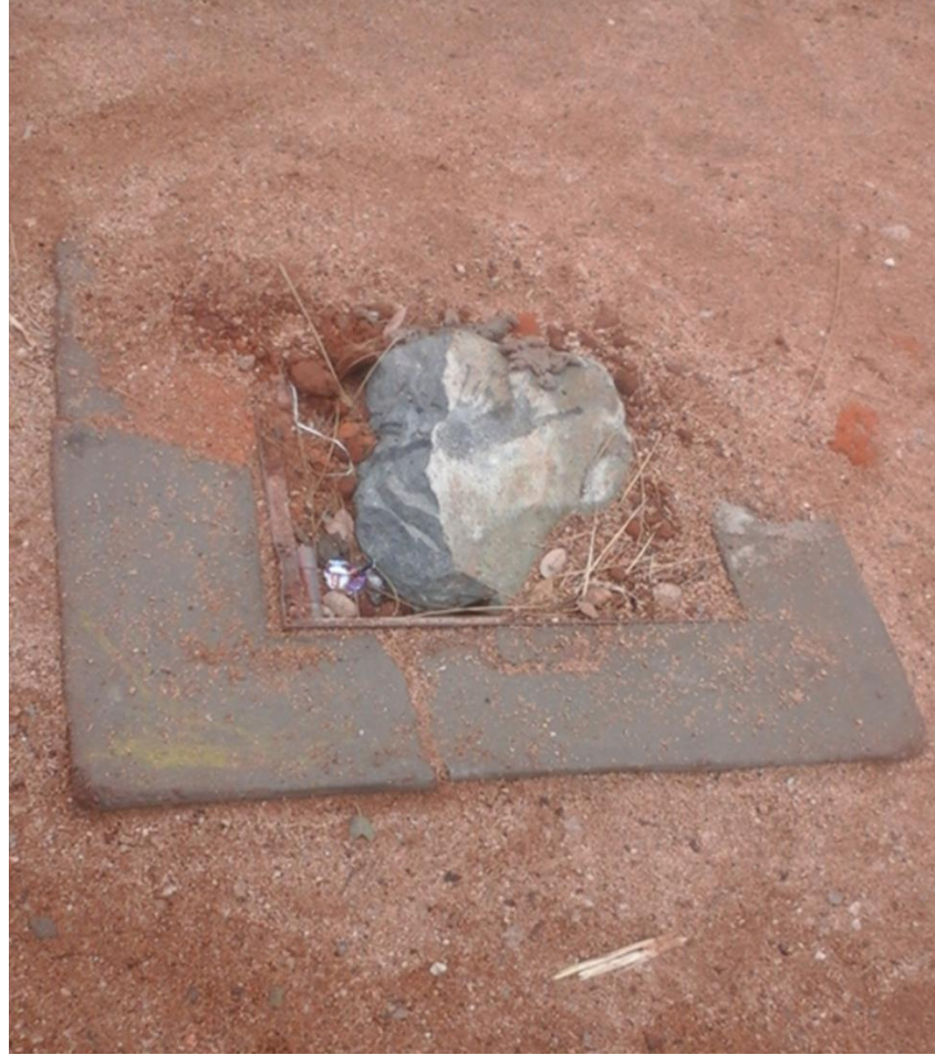
Figure 1 (left). Image of a non-functional groundwater monitoring point in Machinga District. The monitoring point has been vandalised. (ND WASH Consultants, 2017)
