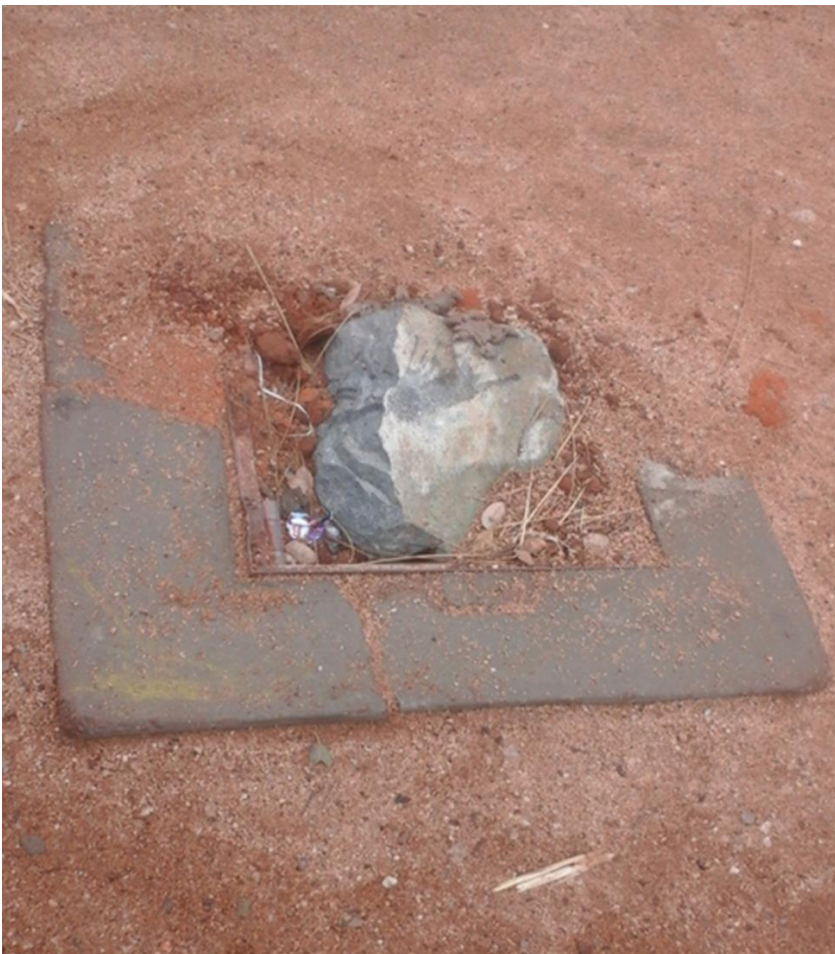
Figure 1 (left). Image of a non-functional groundwater monitoring point in Machinga District. The monitoring point has been vandalised. (ND WASH Consultants, 2017)
